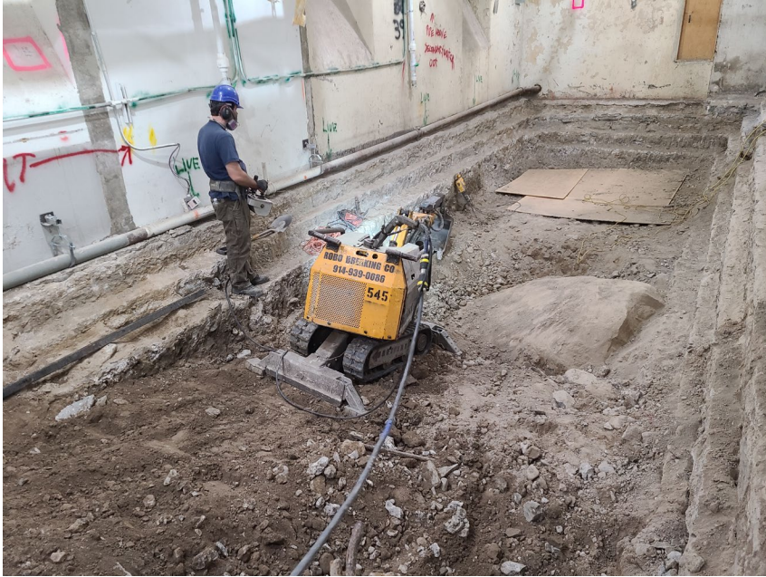
Excavation for elevator and stair
