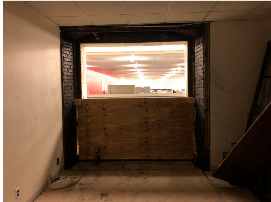
Mezzanine connection to South Court through existing window
