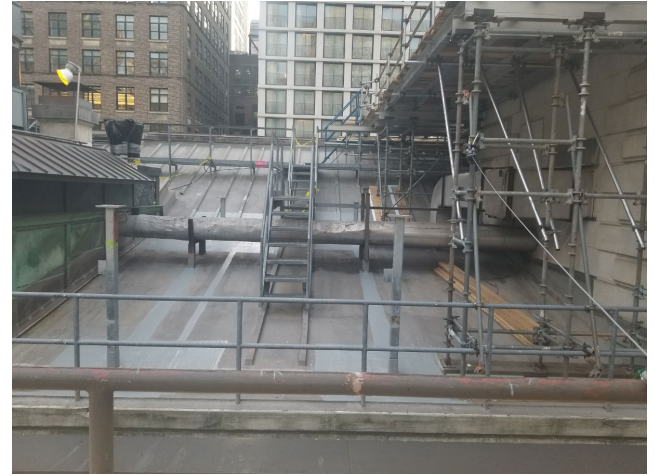
Permanent roofing around posts installed.
