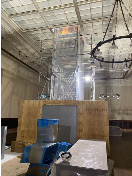
Solomon protection: Air handling units
